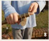
step 8 Continue wrapping around in this direction, whilst keeping the string as taut as possible. Repeat approx 3-4 times. More is fine, or if you're near the end of your string make less turns. Leave about 10cm remaining to tie-off to the loose end left from your initial 'tying on' knot. At this stage, if the lashing has not become taut and the joint rigid, then we suggest you unwrap the frap and re-do it, pulling harder this time.
