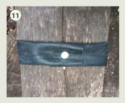
**11.** Cut a length of the bicycle inner tube long enough to wrap around the backplate with some overlap. Wrap the tube around in a position where it will hold the soap bottle firmly against the backplate. Attach it with a clout nail or two. Check the length so that they don't go through the backplate and puncture the soap bottle!
